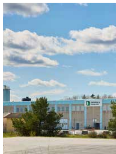
Heidelberg Materials Precast Abetong, Hallstahammar.
