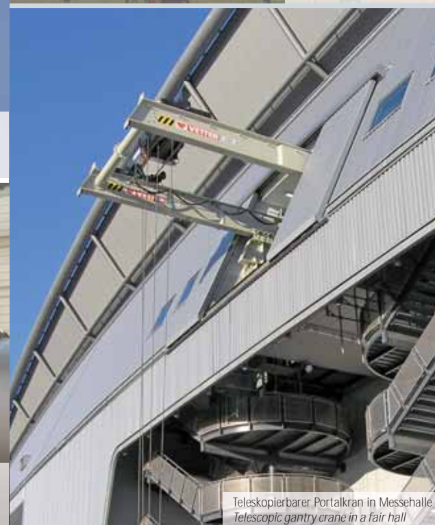
Servicekran in 114 m Höhe Service crane in 114 m height
